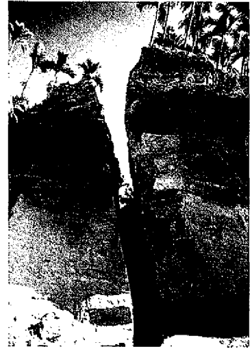
Photo. 11. A deep-seated, opened high-angle joint in the slid rock masses on the northern part.
