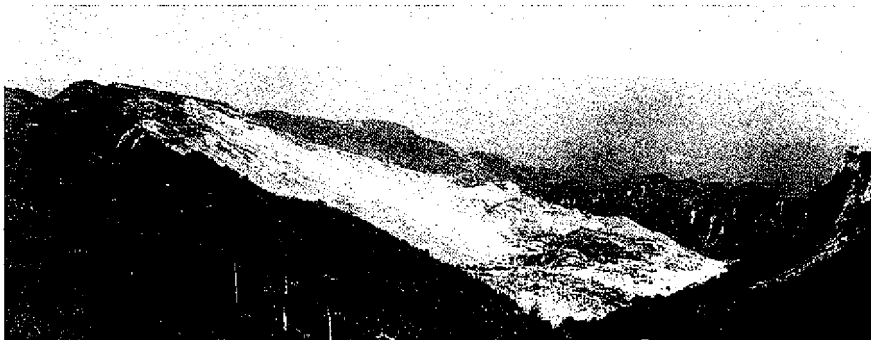
Photo. 1. A distant view of the Chiufenershan landslide from south toward north.
